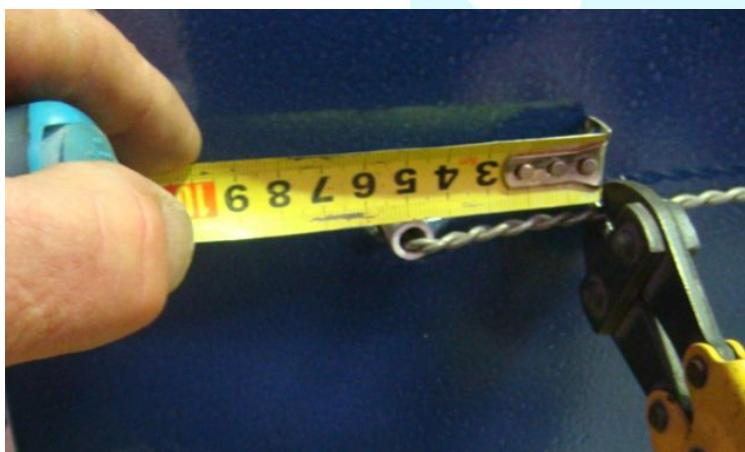
Measure 50mm from centre of bend and cut excess tail off.
